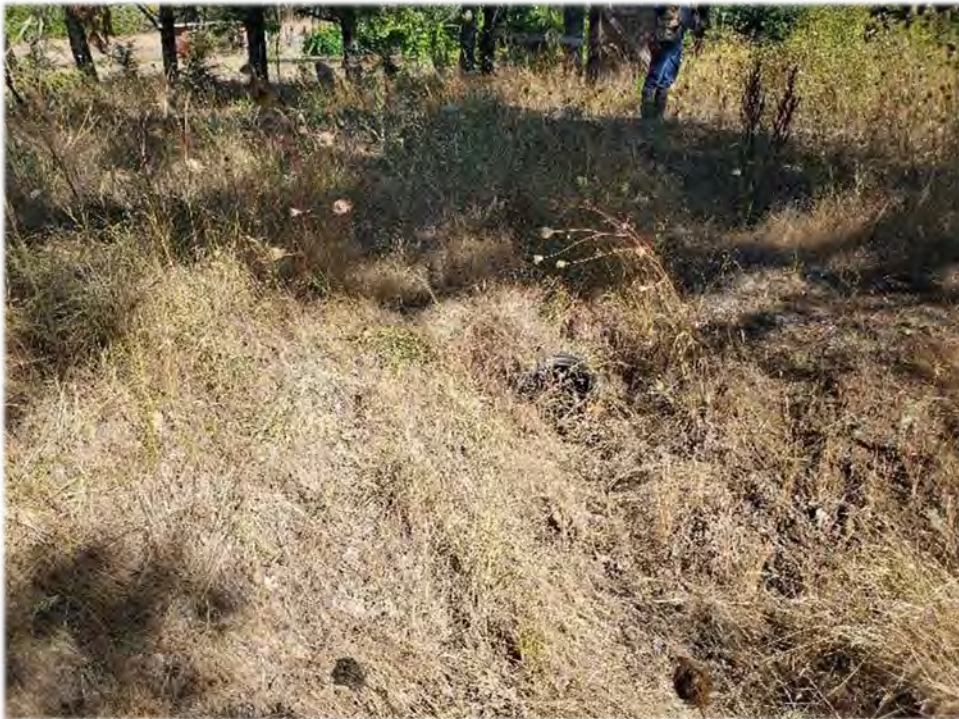
Photo Point 2. Showing culvert along northern site boundary. Culvert extends underground offsite to the north.
