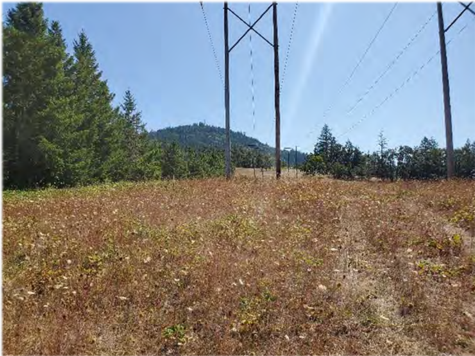
Photo Point 11. Facing east, upslope in powerline right-of-way.
