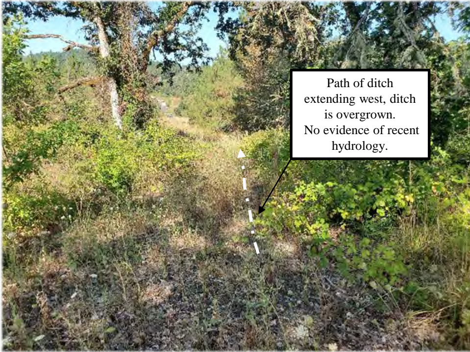
Photo Point 3. Facing west, downslope showing abandoned ditch.
