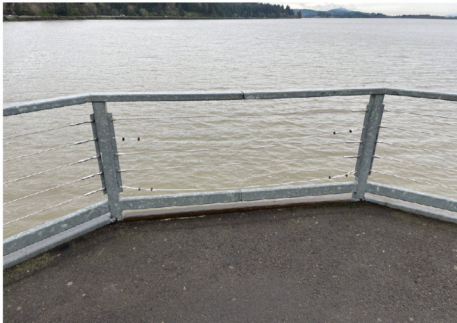
Span 4 Outlook Cable Handrail
