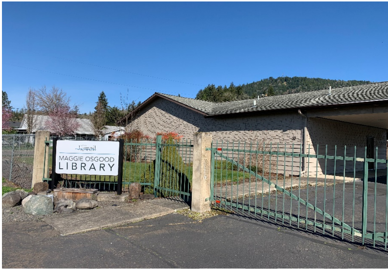
Picture 1: Entryway to existing building
