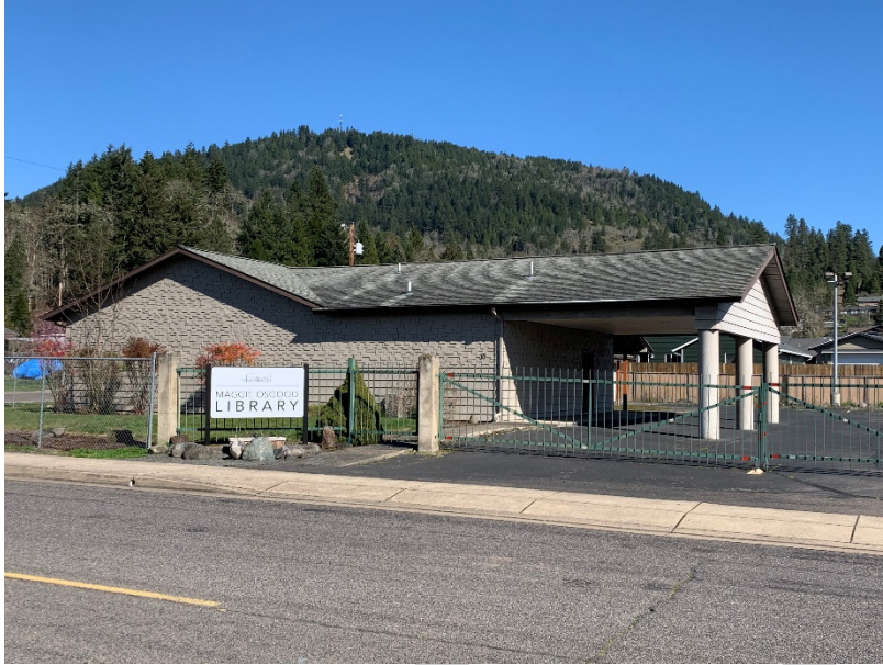
Picture 3: Outside view of existing building
