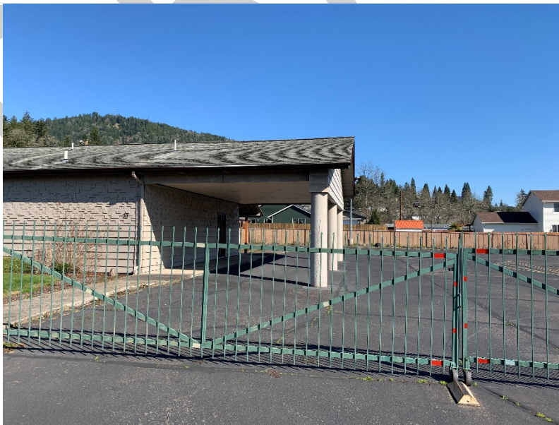
Picture 2: Entryway to existing building
