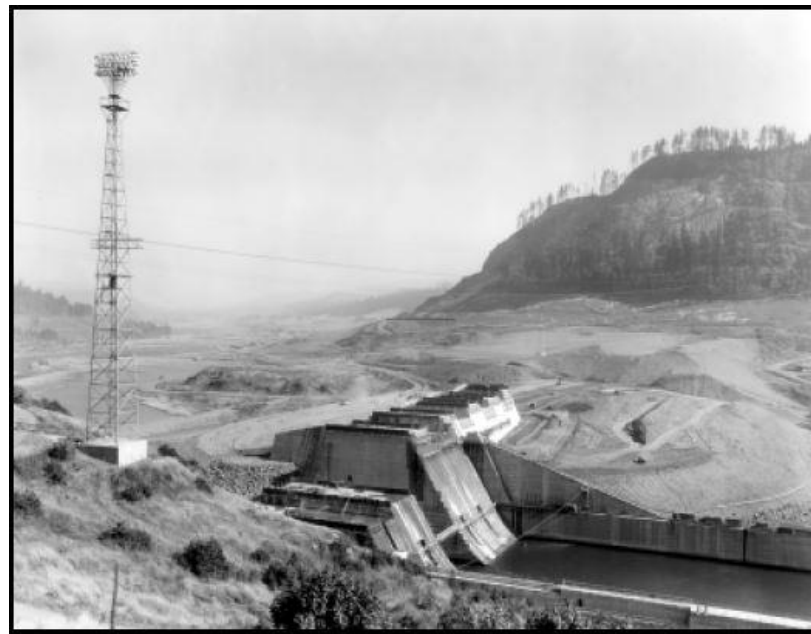
Construction of the dam at Lookout Point, 1952
