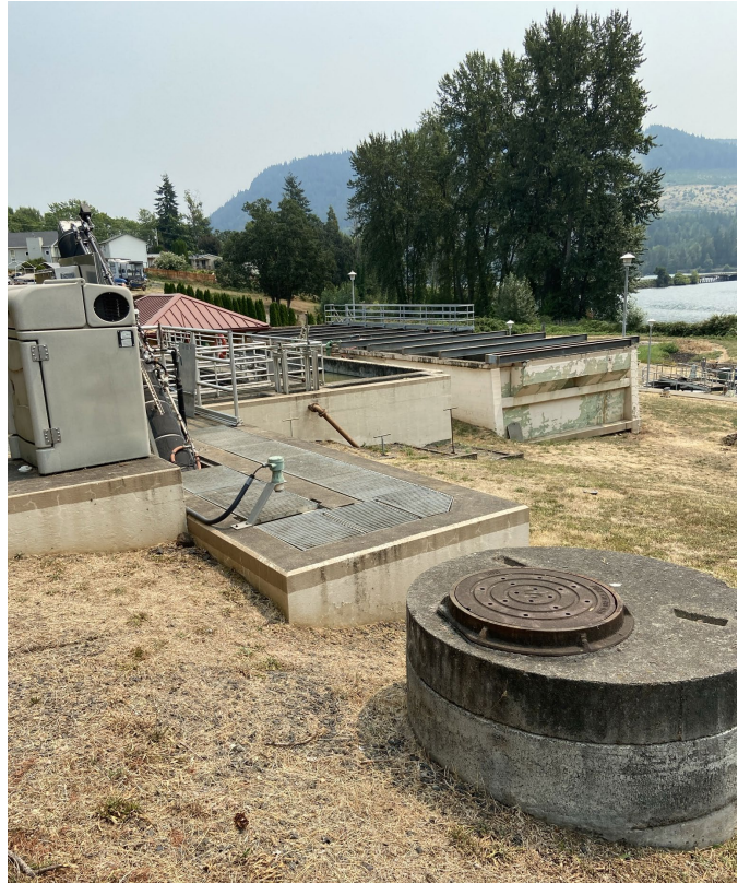
Figure 2-6: Manhole upstream of the WWTP Headworks
