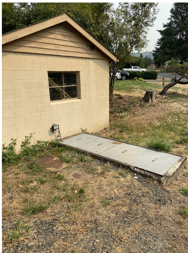
Figure 2-1: Alder Street Pump Station
