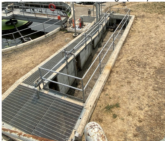
Figure 2-11: Solids Contact Channel
